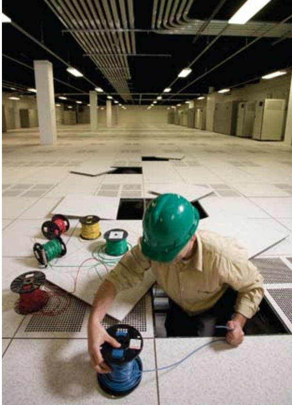
Left: Installing cable under the raised floor of a data center. Right: President Micheal Nicholson P.E and CEO Sean Mulleady standing outside one of their projects dual-feed 26.4 KU/40 megawatt electrical lineup.
